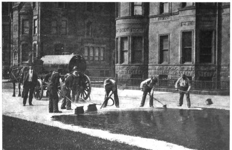
SPREADING TARVIA ON COMMONWEALTH AVENUE, BOSTON.
